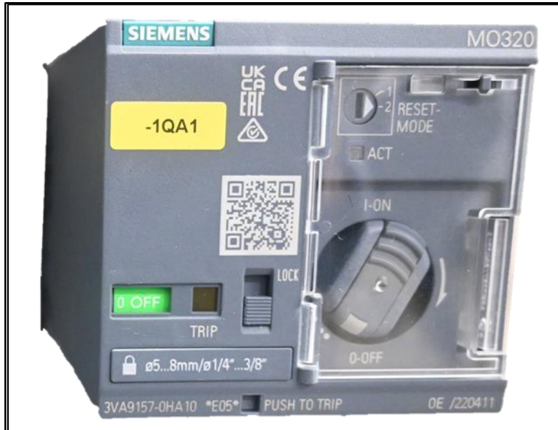
Fig. 13 Power circuit breaker 1QA1 in ControlShield right front
