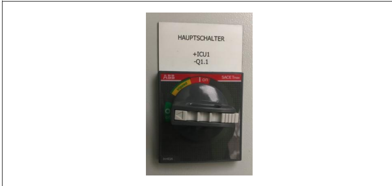
Fig. 5: Main switch on the ICU
